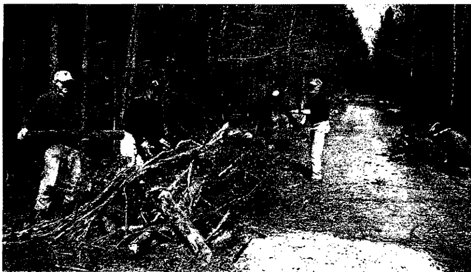
PITCHING IN - TRTC Pres. Bill Bussey, left, gets help from Chris David and Cotten Tyler clearing downed trees from South Durham County section of ATT. Volunteers also are gathering and hauling off truckloads of illegally dumped household trash and construction waste.
