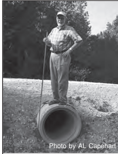
Dunn-Erwin Trail Boss Thomas Jernigan examines upgrade for planned asphalt surface.
